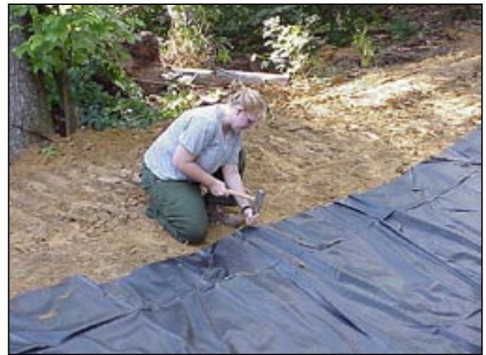
The liner is secured with stakes.
