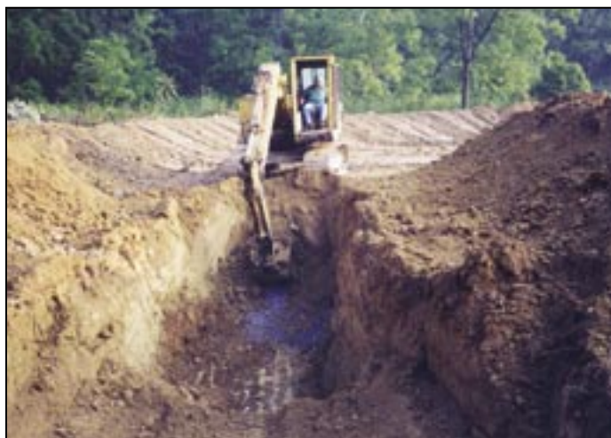
Track-hoe digs a trench down to bedrock to form the core.
