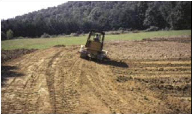
Make gradual slopes on the dam.
