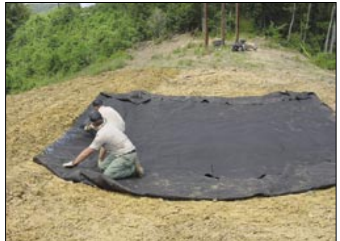
A liner is placed in the depression.
