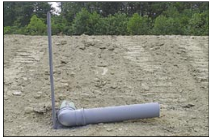
The same pipe can be moved parallel to the ground to drain the wetland.
