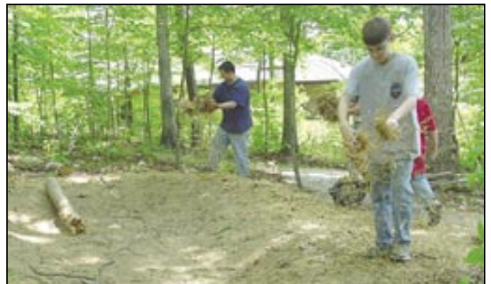
They seeded and mulched the exposed soil.
