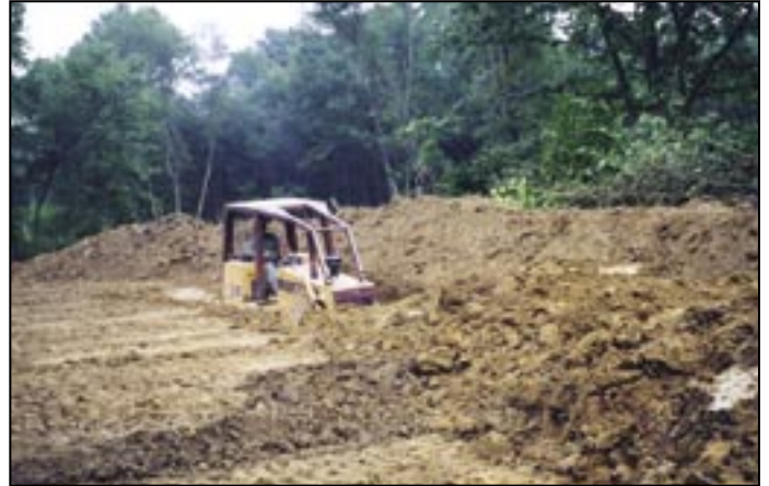
Make a core under the dam location.
