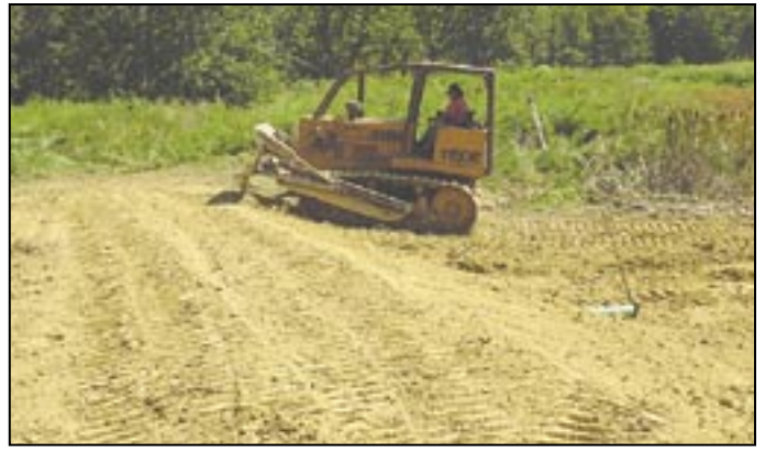
Pack the dam in layers.
