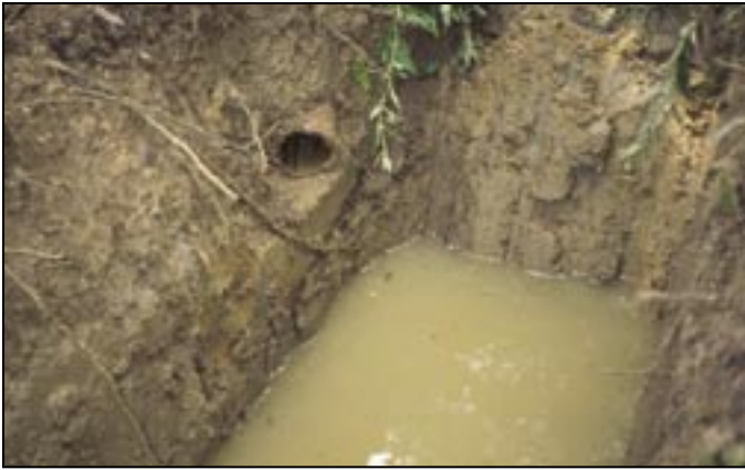
The core will crush buried drainage tiles.
