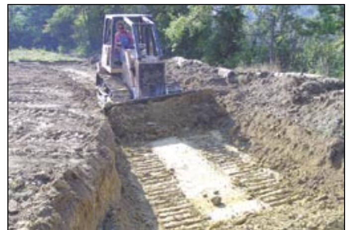
Core is located under the entire dam.
