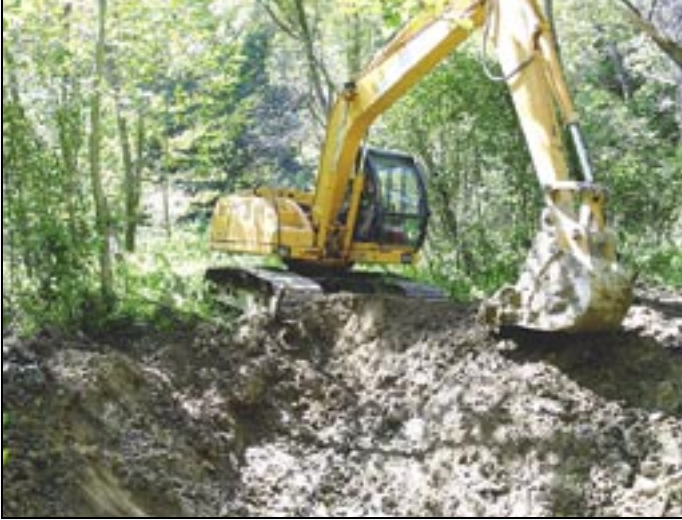
Track-hoe making a vernal pond in a wooded area.
