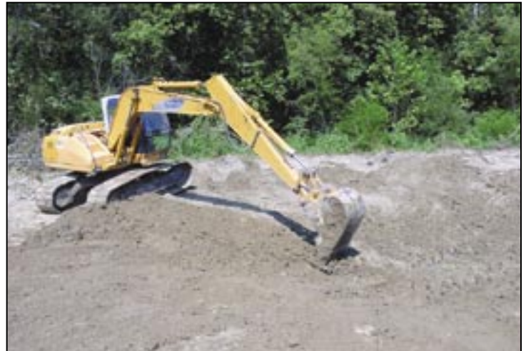
This track-hoe is being used to make an ephemeral wetland. These machines are also used to drain natural wetlands.
