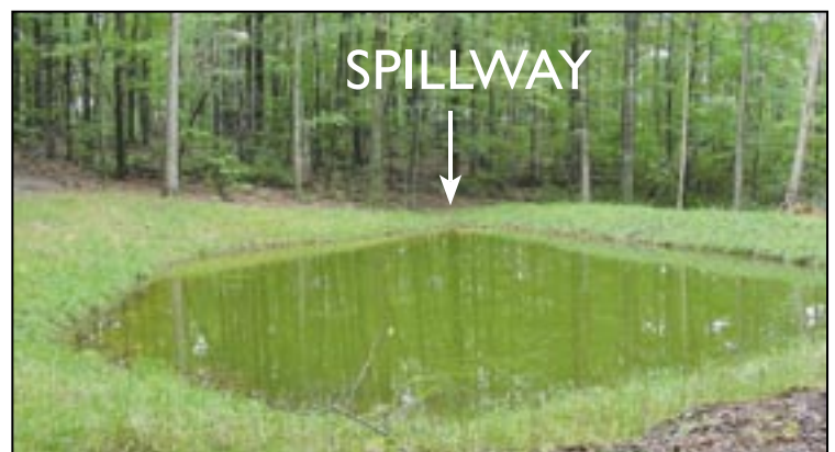
The spillway provides a path for water to leave the wetland.
