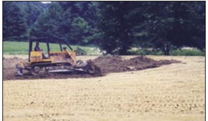
Spread topsoil on the bottom of the wetland.
